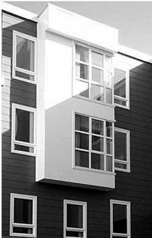
FIGURE 8 Bay windows are a relatively inexpensive means of enlivening facades and bringing light into dwellings.
