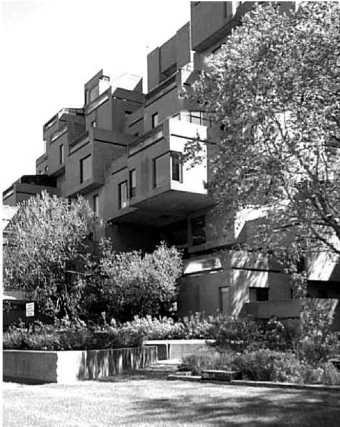
FIGURE 4 Each module of Habitat in Montreal supports several others. The structure needed to support these modules makes the Habitat model more costly than other forms of manufactured housing.
