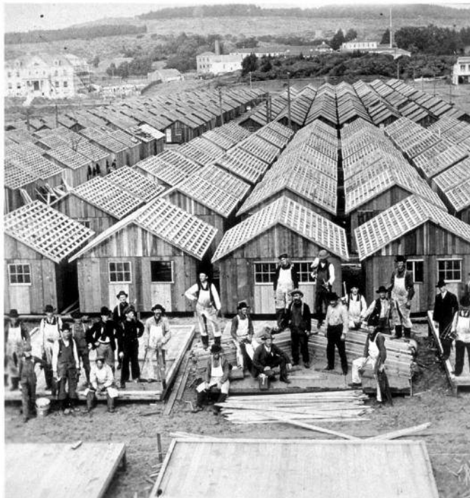
FIGURE 7 Earthquake cottages in San Francisco, ca. 1906. Hundreds of these small dwellings housed those who lost homes in the San Francisco earthquake and fire. Some were later moved to other sites and remain in use today.
