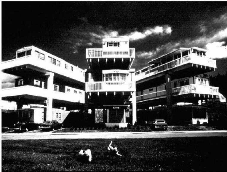
FIGURE 3 Mobile homes are less expensive than construction housing, but their single story limits their use to low-density areas. A few have attempted to overcome this inherent limitation, as in this 1960s demonstration (SkyeRise Terrace by the Frey Building Company), by placing the units onto a concrete support structure.
